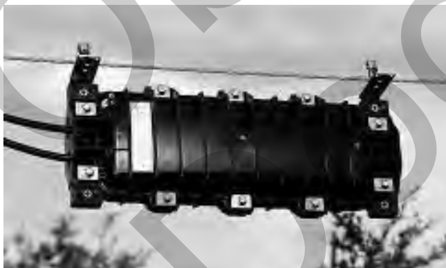
3M™ 2178-S case mounted on strand.
